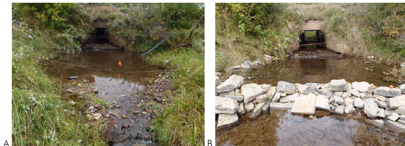
Figure 38. MCE015 before (A) and after (B) Tailwater control weir installation.
