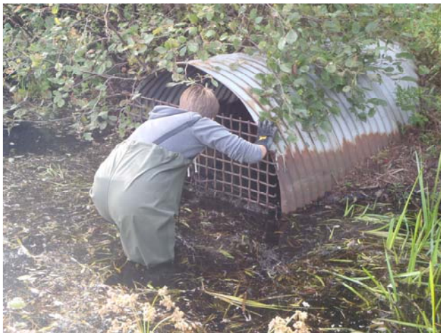
Figure 15. A and B-CARP staff removing debris from inflow debris cage at HEN001.
