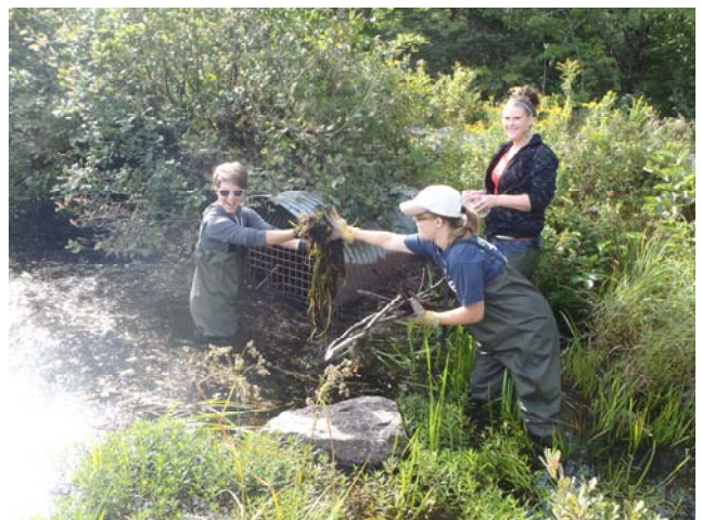
Figure 15. A and B-CARP staff removing debris from inflow debris cage at HEN001.
