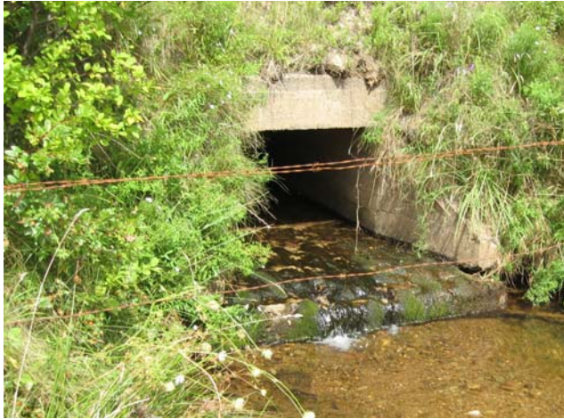
Figure 40. MCE015 Outflow before (A) and after (B) Tailwater control weir installation. NOTE: Photo A was taken in summer 2010 and photo B was taken October 2011, one month after weir installation.
