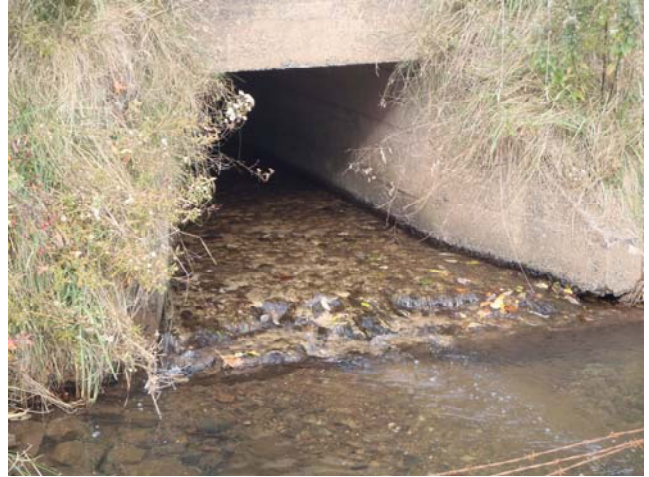
Figure 40. MCE015 Outflow before (A) and after (B) Tailwater control weir installation. NOTE: Photo A was taken in summer 2010 and photo B was taken October 2011, one month after weir installation.
