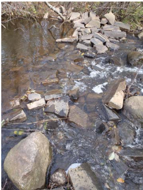
Figure 35. Weir A after extreme rain storm.
