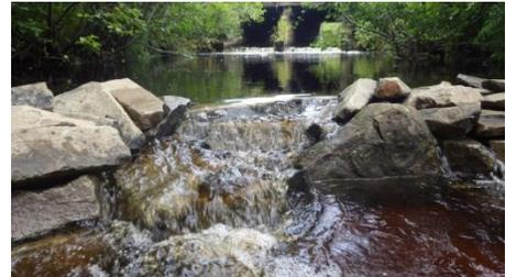
In order to address habitat fragmentation caused by previously identified barrier culverts, fish passage remediation actions were completed. These actions included the installation of tailwater control structures, baffles, and outflow chutes.
