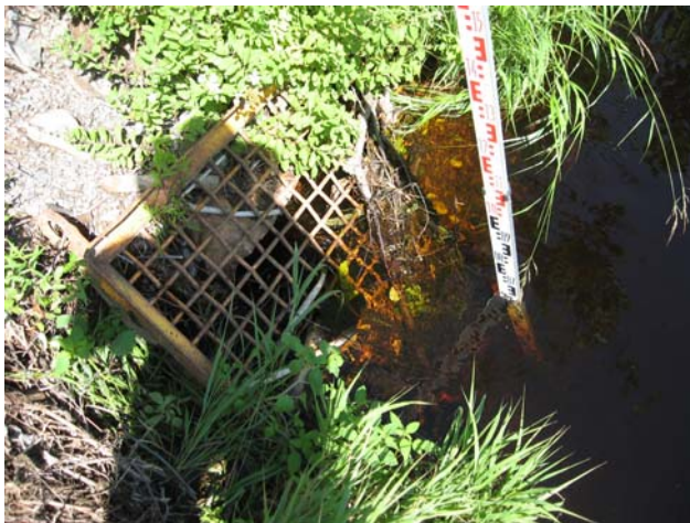
Figure 11: JTM001 Inflow with debris cage
