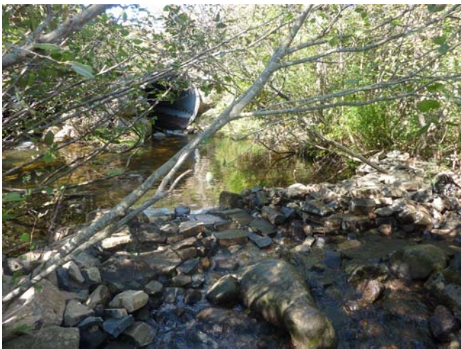
Figure 45: Rock weir following its installation
