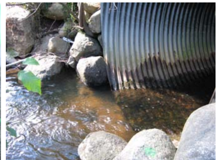
Figure 51: Culvert #1 after tailwater Control
